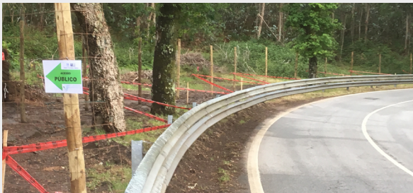
Good tape and tempory fencing to keep spectators at a safer distance
