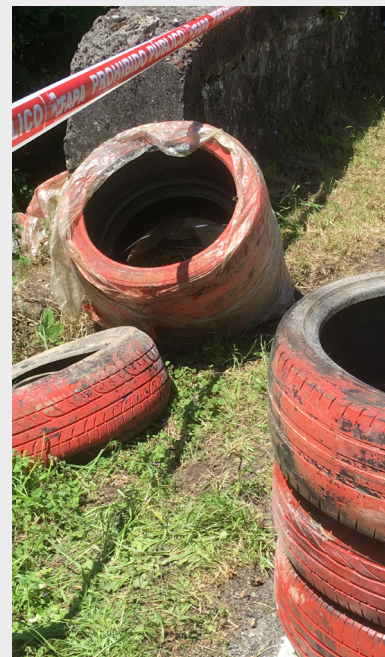
Poorly positioned and constructed tyre stack
