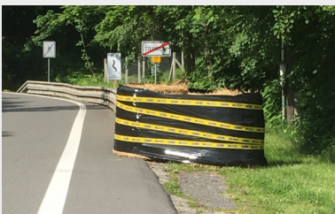
Good use of Straw bales to protect dangerous point
