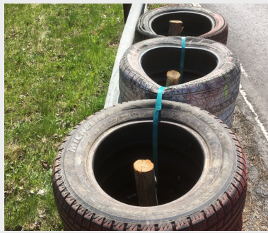
Tyre stack well constructed
