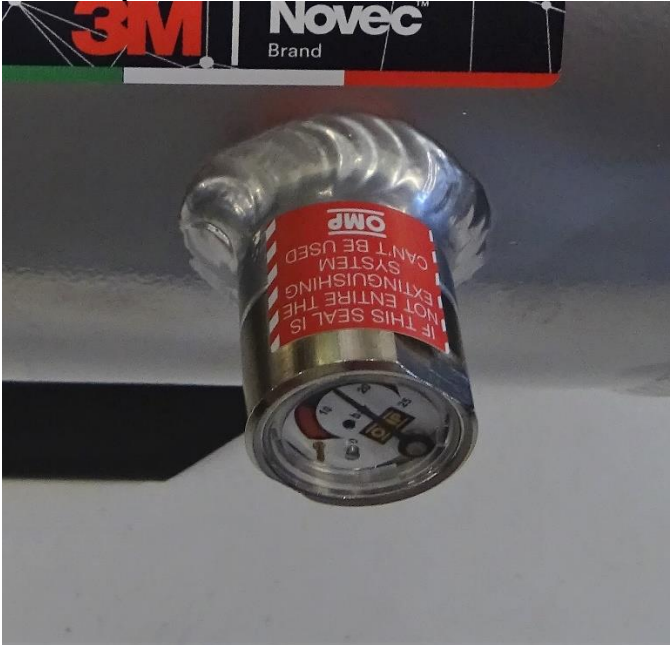
Fig. 3 Pressure gauge tamper proof seal
