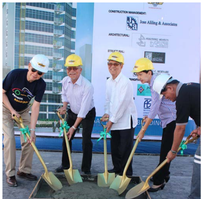
The AAP recently held the topping off ceremony of its new 10-storey building in Quezon City, headed by (left to right) APP Directors, David Arcenas, Augusto Lagman, Jacinto Mantaring, Aida Sevilla-Mentoza, and AAP Lingkod’s General Manager Jose Mundo.
